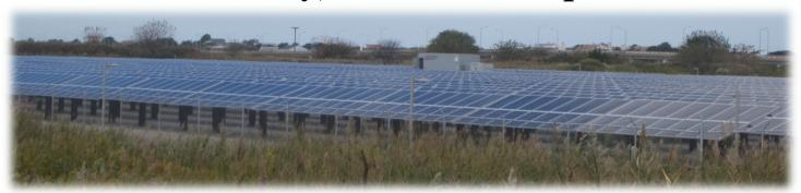
The expansive solar array visible when traveling east bound on the Hampton Roads Bridge Tunnel is, by far, the largest in the Commonwealth. Rated at 2.1 MW the Monkey Bottom installation at the Norfolk Naval Station consists of over 8,000 panels covering 10 acres. The system went online at the end of 2012 and provides about 2% of the Naval facility's power. Bay Electric of Newport News installed the American made SolarWorld Panels with design assistance from the Blue Sky Group, of Venice, FL.
