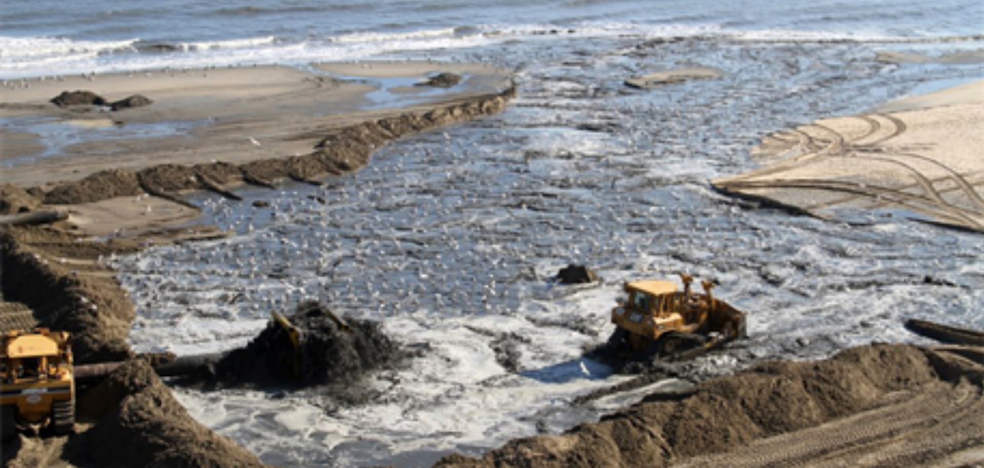
Beach Replenishment Project, Virginia Beach – Cost $13.7 million – Image: US ACOE
