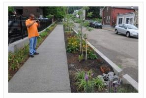
Greenfield uses pervious concrete, garden to capture and purify water
